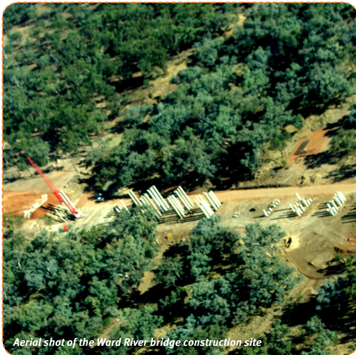
Construction on the new Ward River bridge
